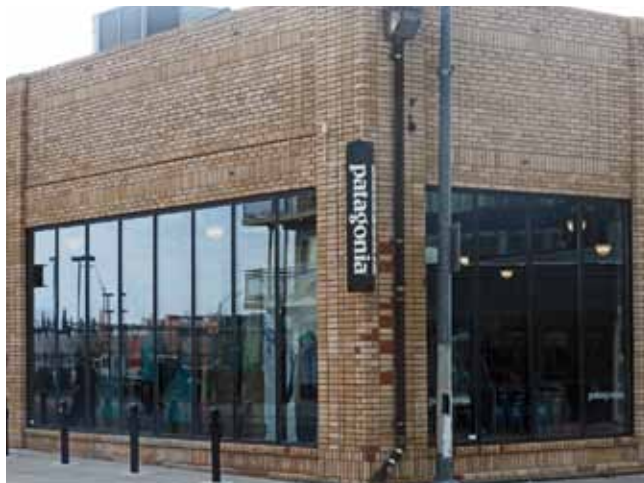
130 S. Center Street, built in the 1940s for the Hudson Motor Car Company, now the home of Patagonia.
