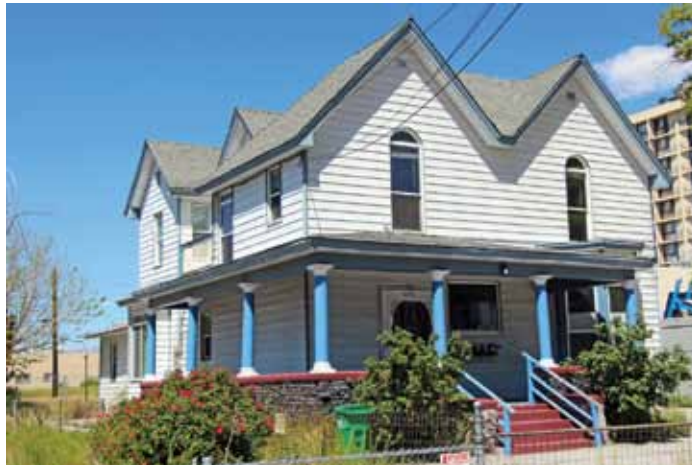
The Bender House, c. 1877. Originally built as a Gothic Revival, though the porch with its columns and other additions modified its style. Built for the Bender family, significant early Reno residents whose descendants still live in the area.
