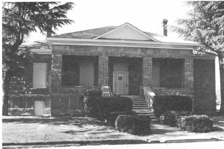
The so-called Stone House, built in 1890 with stones from the abandoned state prison wall (1890 to present). Photo courtesy of Kim Henrick.
