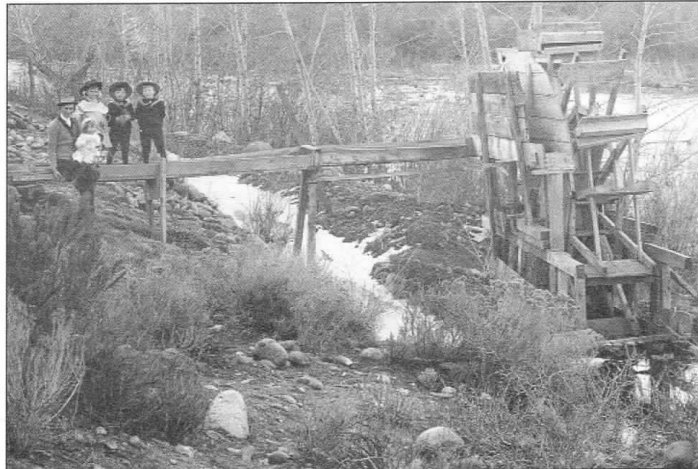
The baby is Elliott Cann, with brothers and sisters. The water wheel and pipe system brought water to their home from the Truckee.
